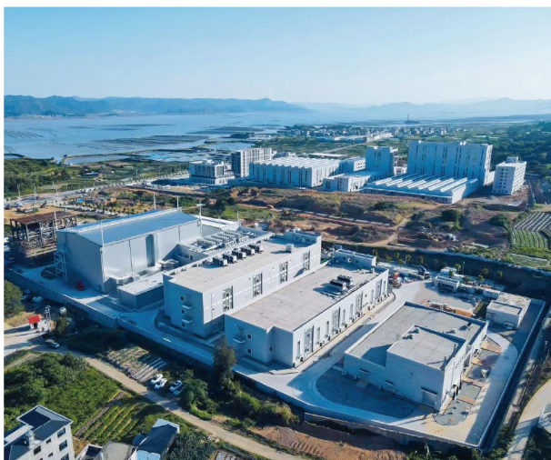
State Grid-CATL Ningde Xiapu 100MW/200MWh Energy Storage Plant, Fujian, China
