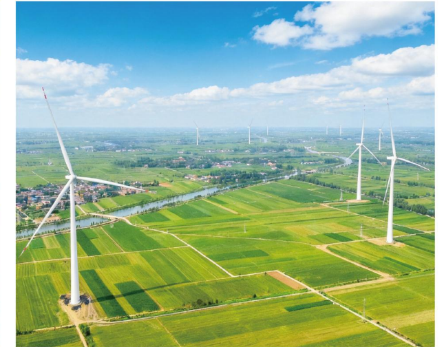
CGE Jingxiang 210MW Onshore Wind Power Project, Shandong, China (EPC)
