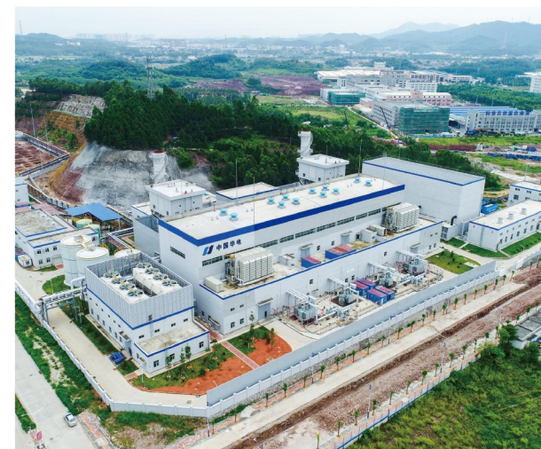
Huadian Jiangmen Combined Cooling Heating and Power Project, Guangdong, China
