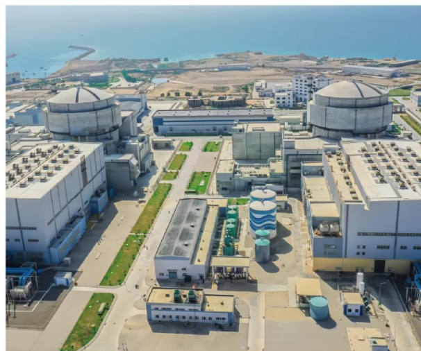
Karachi K2/K3 Nuclear Power Plant Conventional Island BOP Project, Pakistan
