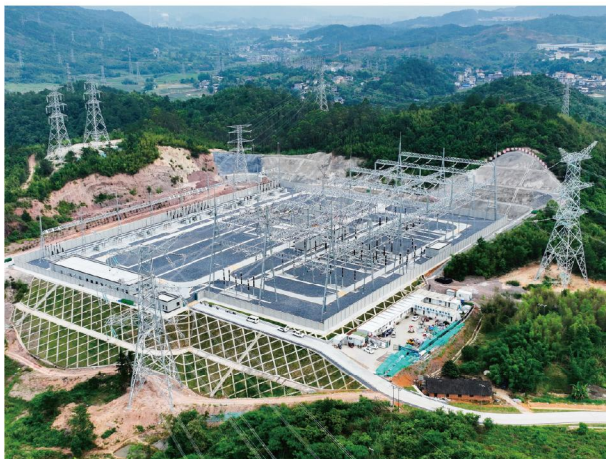
Taoyuan 500kV Power Transmission Project, Fujian, China
