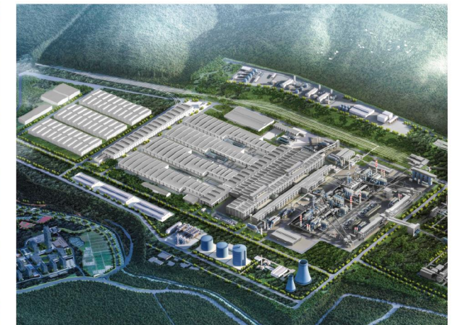
Yukun Steel Plant TL & Substation Project, Yunnan, China (EPC)
