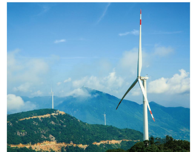
70MW Gaoyushan Wind Farm Project, Fujian, China (EPC)
