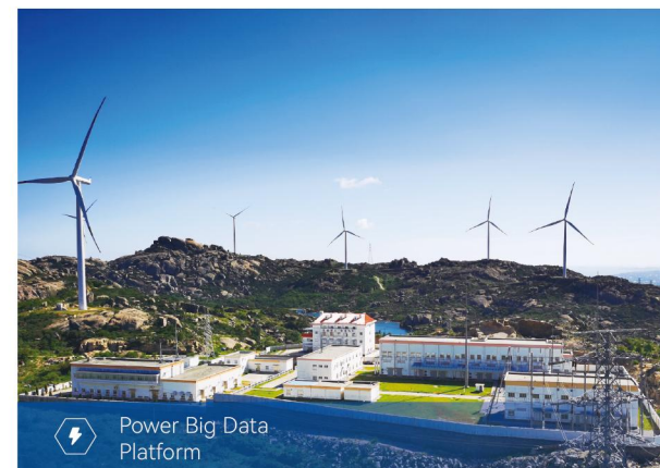
CHN Energy Yanqian Monitoring System for Centralized Control Center Upgrading and Renovation Project, Fujian, China
