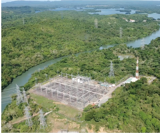
NGCP 230kV Lumban Substation Main Transformer Upgrade Project, South Luzon, the Philippines (EPC)
