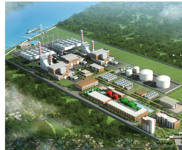
Lupsha 800MW CCGT Power Plant, Bangladesh
