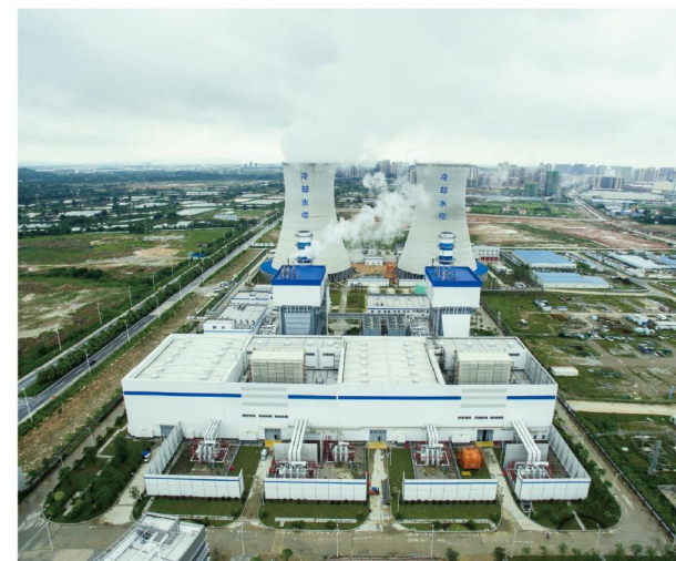
Sihui 2x400MW Combined Cooling Heating and Power Project, Guangdong, China
