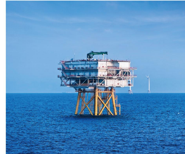
220kV Offshore Substation of Qingzhou IV Offshore Wind Power Project, Guangdong, China
