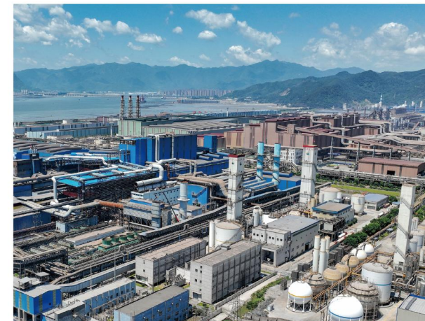
Minguang 220kV Power Transmission and Substation Project, Fujian, China (EPC)
